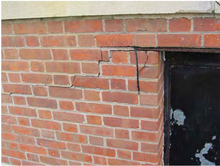
Cracks noted in exterior brickwork
