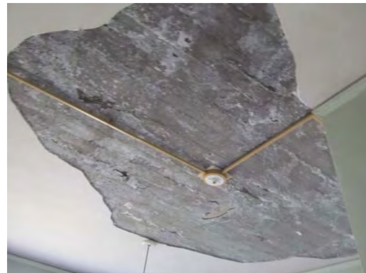
Ceilings at space on third floor level also exhibit signs of moisture infiltration and damage
