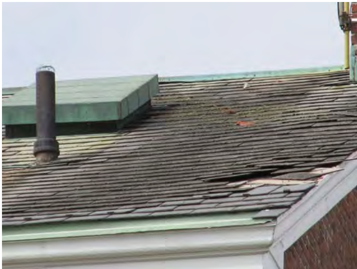
Loose/missing slate roof shingles
