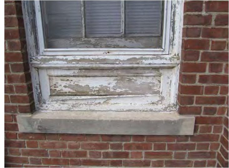
Typical condition of wood trim and paint finish at windows
