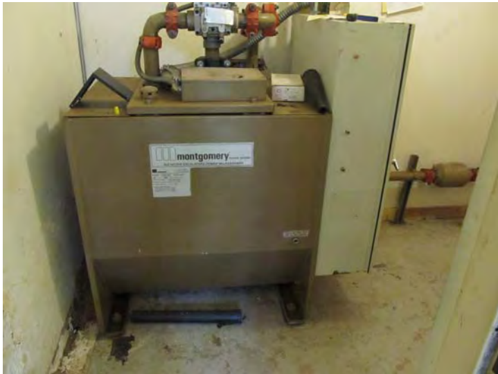
Hydro-mechanical and controller/dispatcher equipment for elevator has been offline for an extended period of time
