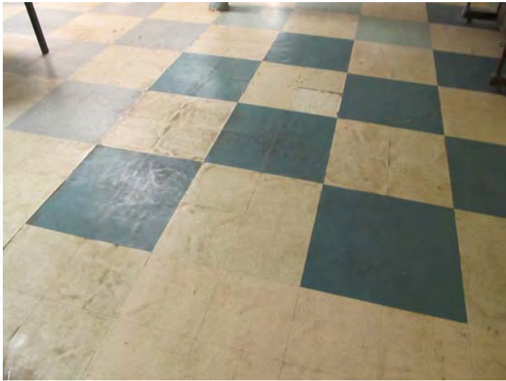
Vinyl flooring in multi-purpose/dining room is worn/damaged and in need of replacement
