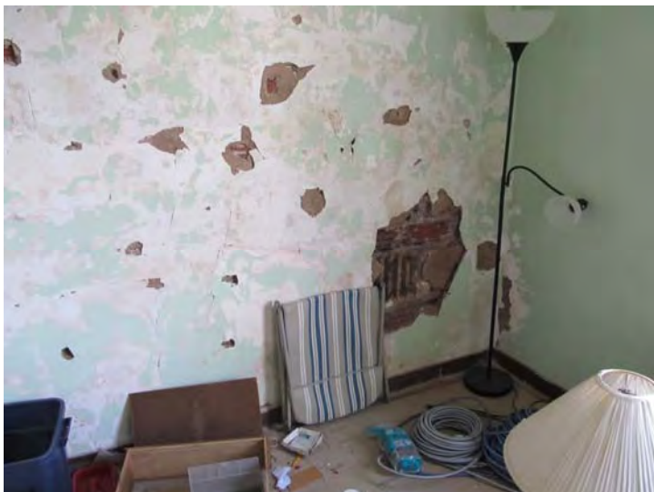
Wall surfaces at unused space on third floor level of building exhibit signs moisture infiltration and damage
