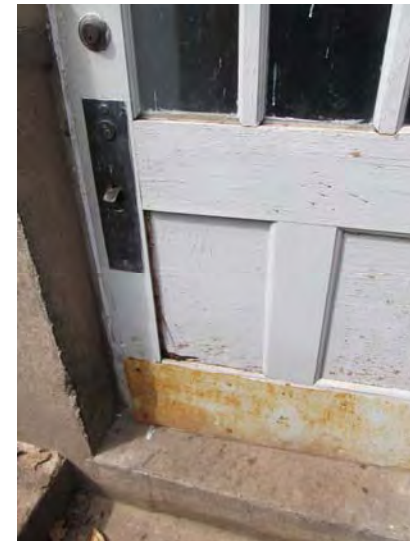
Wear/deterioration on entry door to lower level of building
