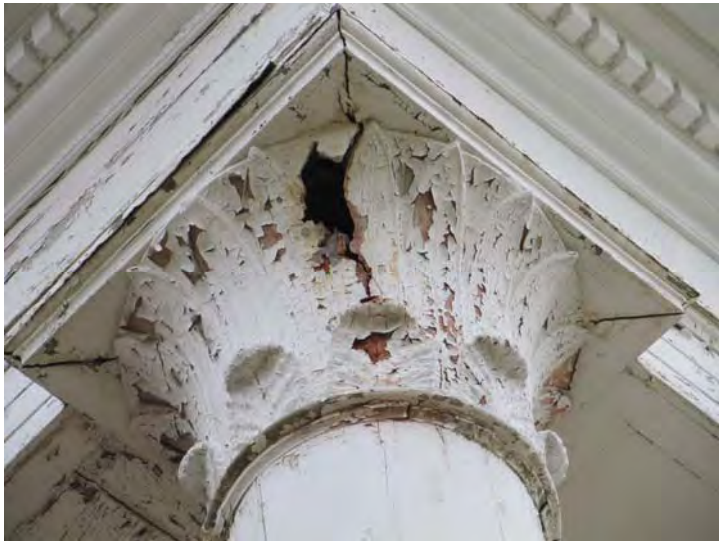
Decorative capitals at top of columns exhibit varying levels of deterioration
