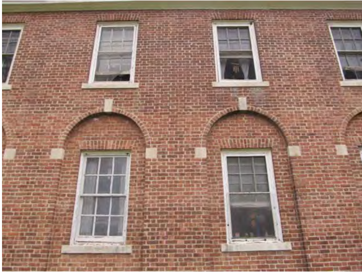
Original, wood-framed, single-glazed, windows are typical throughout the entire building
